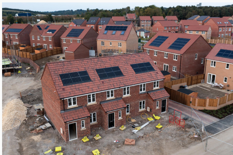
The roof of a new build house with integrated solar panels under construction
